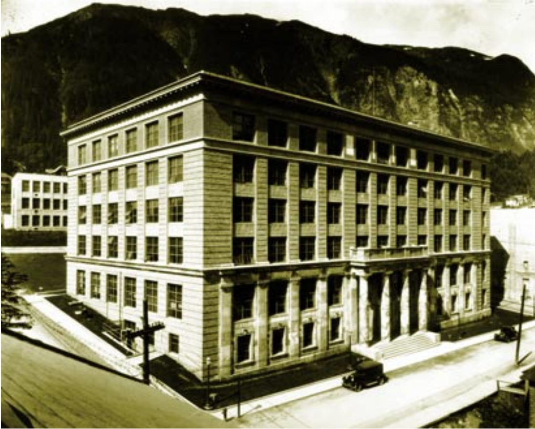
Construction of the Territorial Capitol was completed in 1931. Alaska's collections of books, manuscripts, natural history, and cultural artifacts were displayed on the second floor until the new Alaska State Museum was completed in 1967.
